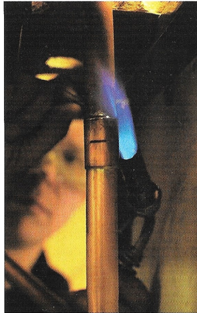
⊙ Copper pipe being worked
