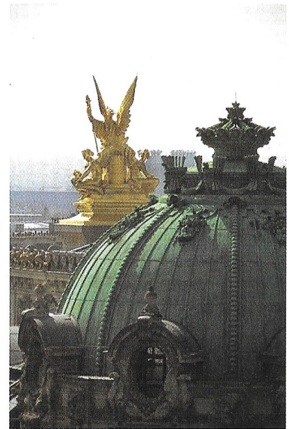
⊙ Oxidated copper turned green on the domed roof of this building
